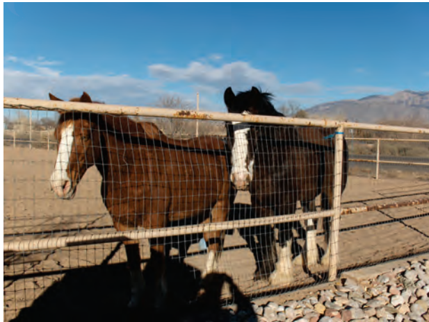
7. Steel pipe with Vermin Wire – Acceptable only on horse corral
